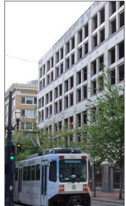
Pioneer Place Garage, Portland, Oregon
