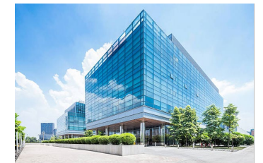
Office Block Building
