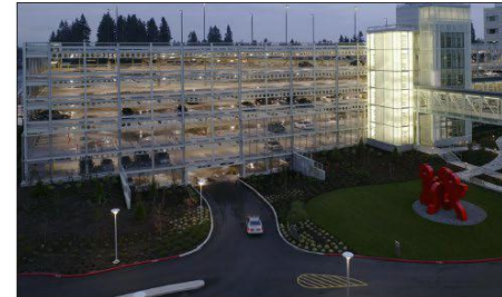
Legacy Hospital Parking Garage, Portland, Oregon
