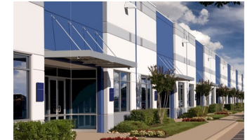
Flex Use Building
