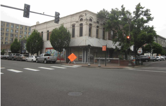
OVERVIEW OF SUBJECT PROPERTY, FACING NW FROM MAIN STREET
