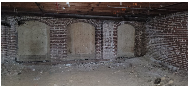
Photo looking to the east of basement walls with openings and plywood.
