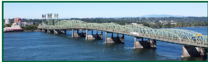
108-year-old I-5 Bridge.
