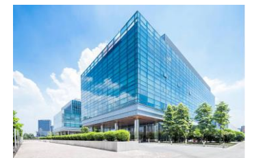
Office Block Building
