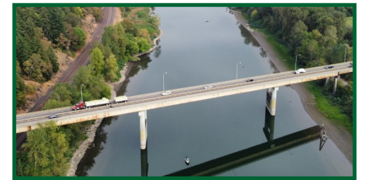
60-year-old West Camas Slough Bridge.
