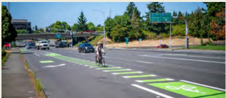
MILL PLAIN AT FORT VANCOUVER WAY
