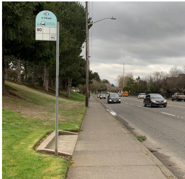
Photograph 2-17. Bus Stop Lacking a Shelter
