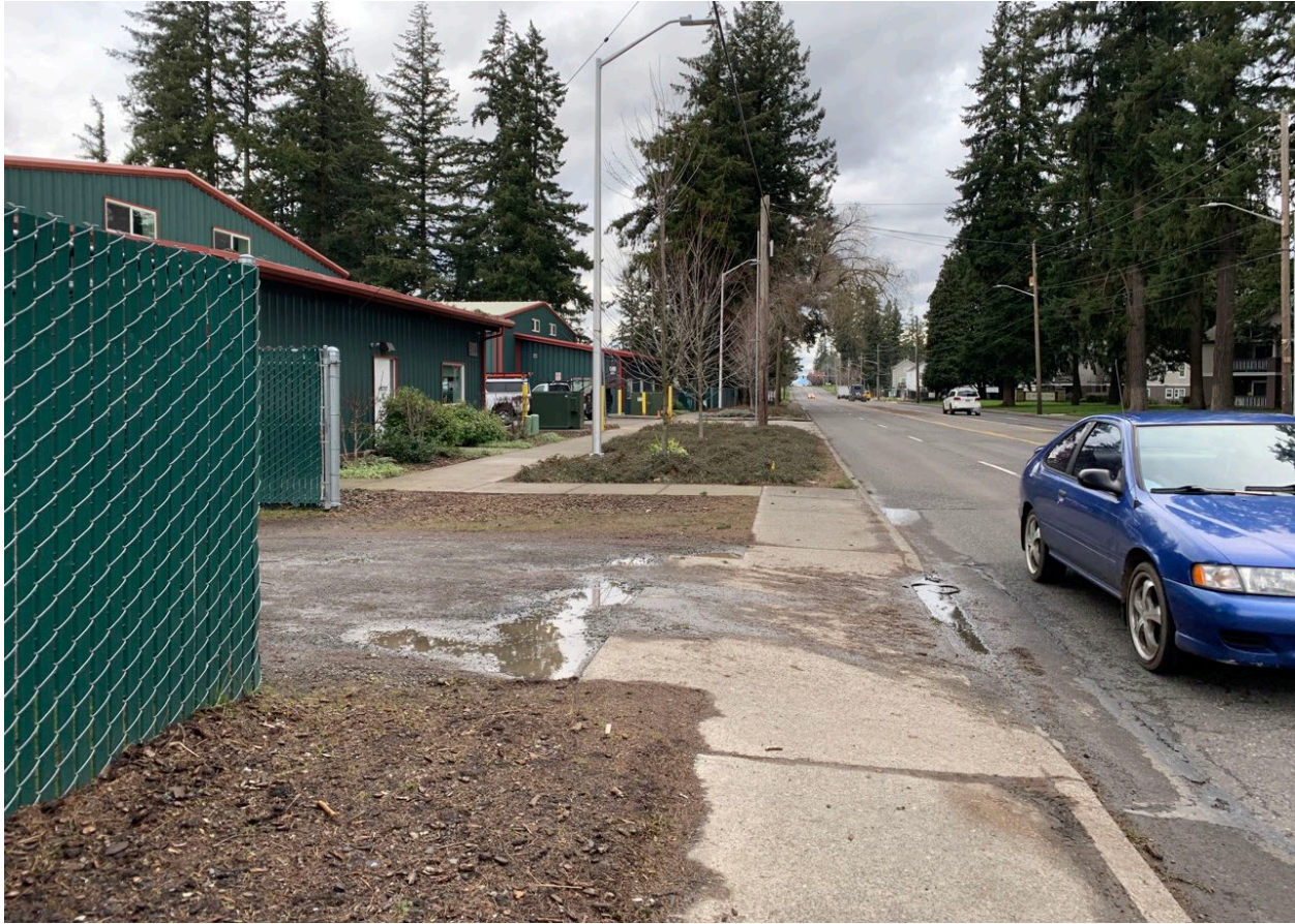
Photograph 2-5. Segment 2: Sharply angled sidewalk configuration (looking north)
