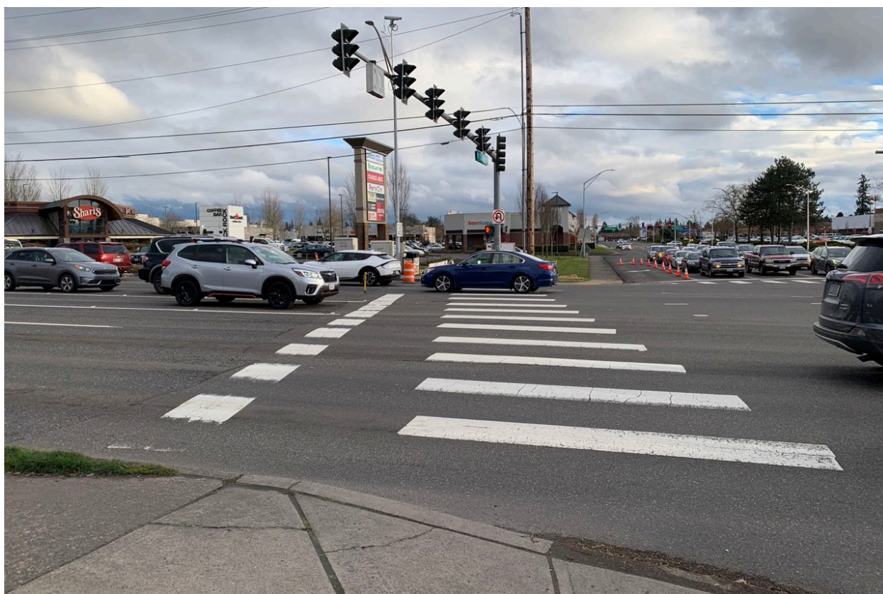
Photograph 2-2. Segment 1: Mill Plain Boulevard Intersection (looking south)
