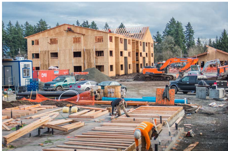
Zone change policy supported K West (above; currently under construction) and proposed Veteran's Village project
