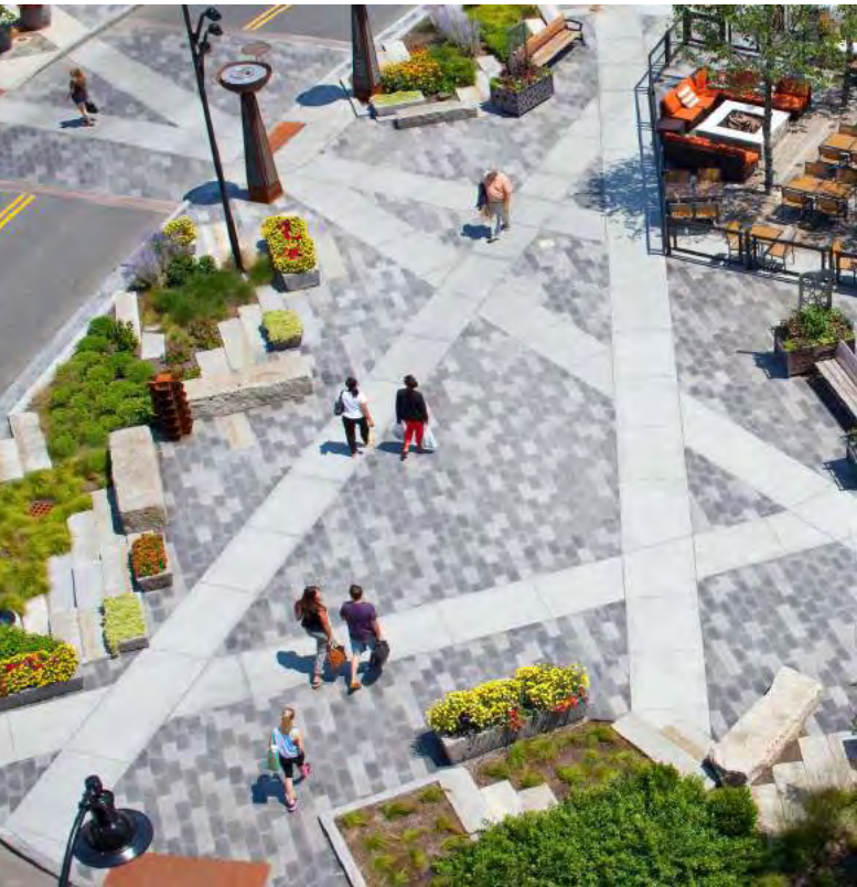
BRICK PAVING + CONCRETE BANDS (LOWER PLAZA)
