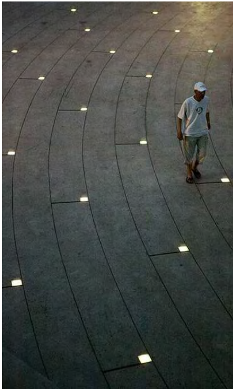
SOLAR LIGHTS IN PAVING
