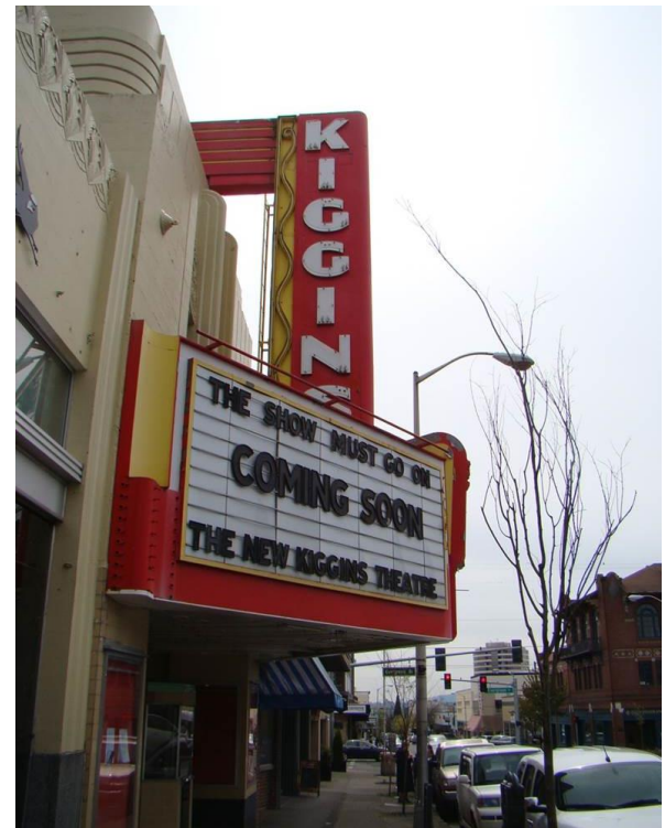
Kiggins Theatre, Vancouver, Built 1936
