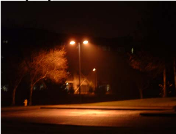
City Hall parking lot light with a fully shielded fixture. This light emits no uplight as evidenced by the downward angle of light seen on the adjacent trees.
