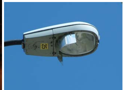
Shield for Streetlight Olympic Way NW (Olympia)
