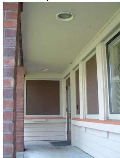
Fully shielded flush mount walkway lights at Tumwater City Hall
