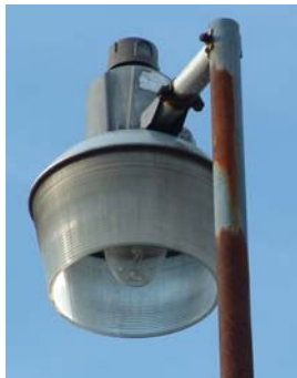
Mercury vapor lamp (Point Tavern)
