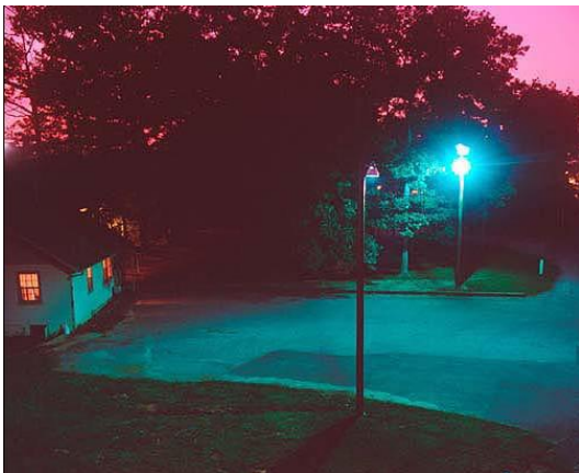
Unshielded yard blaster (far side of street)
