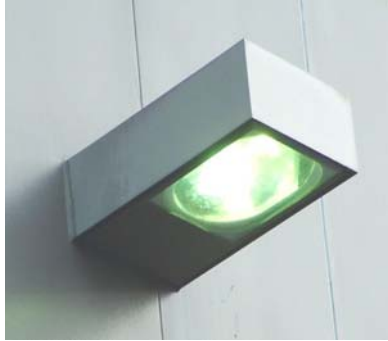
Good: Fully shielded wall box WA Dept of Printing (New Market St.)
