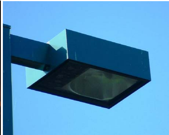
City Hall parking lot light with a fully shielded fixture. This light emits no uplight as evidenced by the downward angle of light seen on the adjacent trees.
