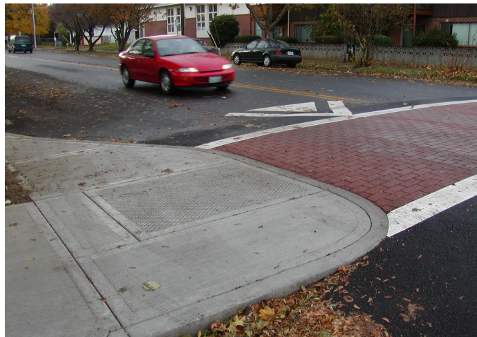
FIG. 53: RAISED CROSSWALK WITH CURB EXTENSIONS
