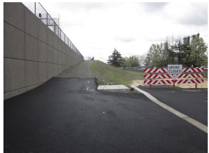
STREET SCENE: FACING EAST ALONG CASCADE STREET TOWARD SUBJECT
