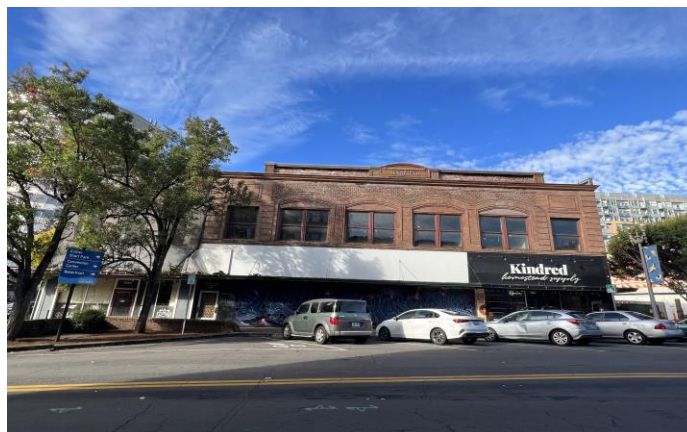
Main Street elevation- Picture date 10/25/2024
