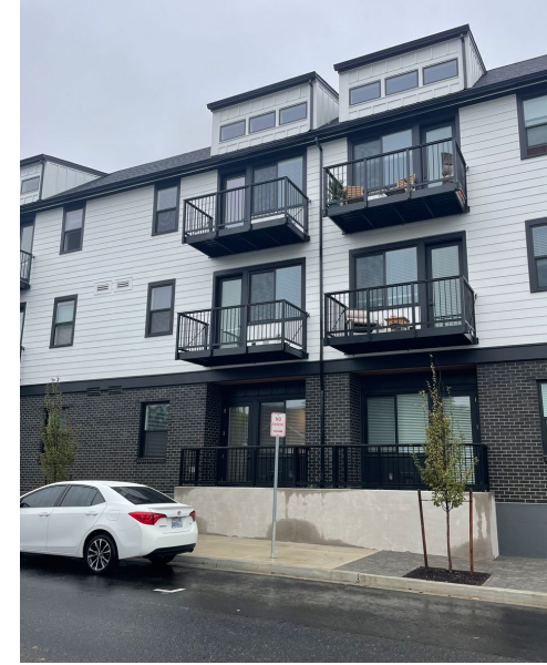
Fiber Cement Siding
