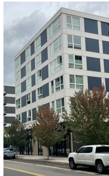
Buildings with Flush Windows
