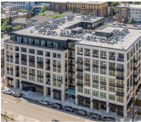
Example of facade with single major break.
