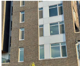
DO Have windows that may be flat or "flush" with facade, if applied to a portion of a building that is part of a façade recess/inset.
