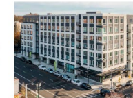
Example with two modulations that break the facade into three distinct massing elements. The breaks are emphasized with a change in color and material. Modulation and articulation of the ground floor complement and align with upper floors.
