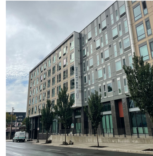
Buildings with Stucco and Fiberboard Cement Panels as Primary Façade Material
