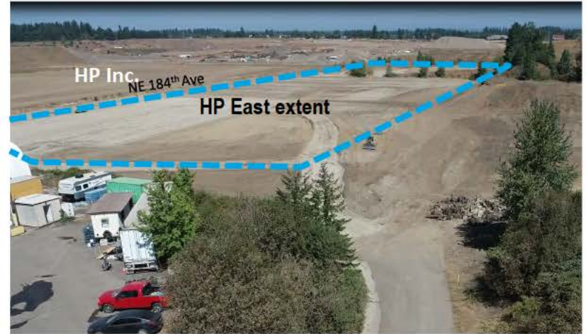
FROM SOUTHEAST CORNER OF PROPERTY LOOKING NORTHWEST
