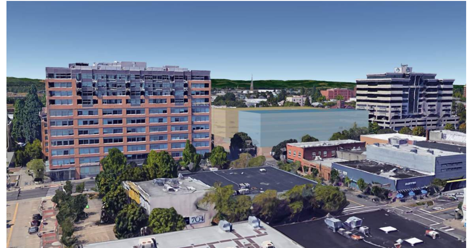
Looking North West
