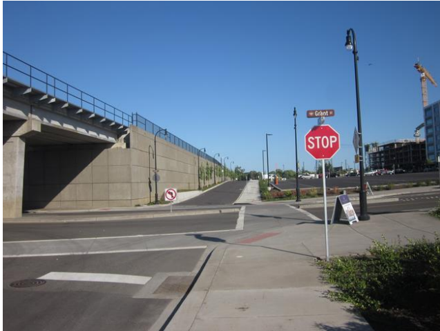
STREET SCENE: FACING WEST ALONG CASCADE STREET FROM GRANT STREET
