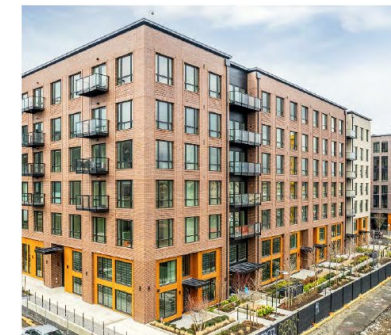
Example of facade with 2 modulations.
