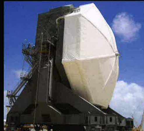
SBX transmission platform interior transmitter.
