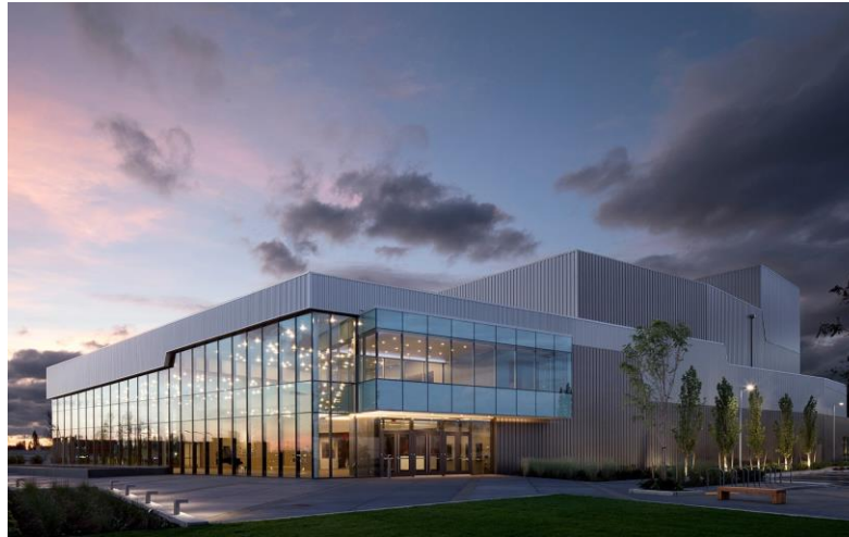
700 seats Federal Way Performing Arts Center Federal Way, WA
