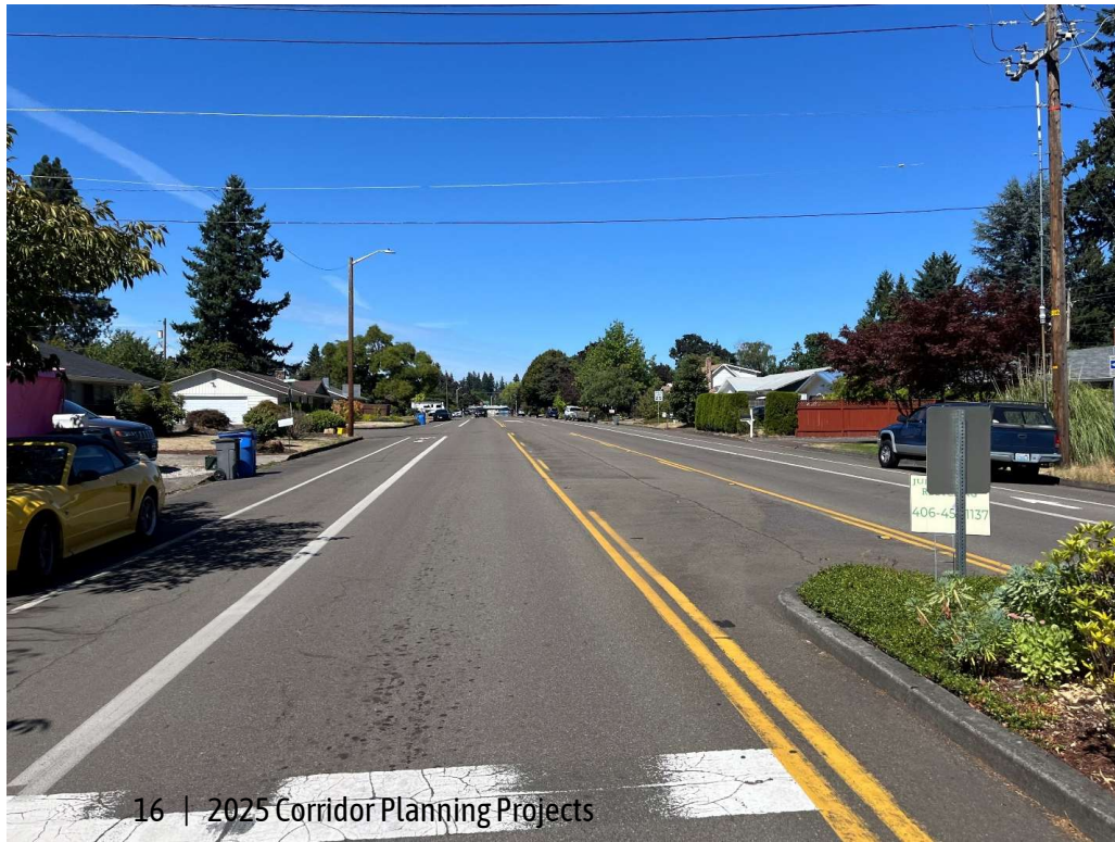
SE 98th Ave at St Helens Ave
