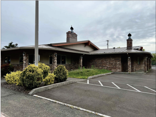
PHOTO 2- SW CORNER OF EXISTING BUILDING
