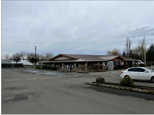
PHOTO 1- NW CORNER OF EXISTING BUILDING
