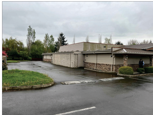
PHOTO 3- NE CORNER OF EXISTING BUILDING
