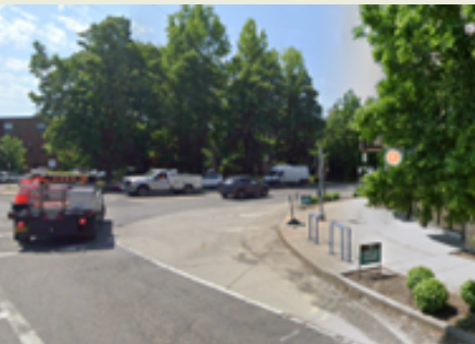
Mountable corners slow down passenger vehicles but can be mounted by trucks. Photo: Google Street View
