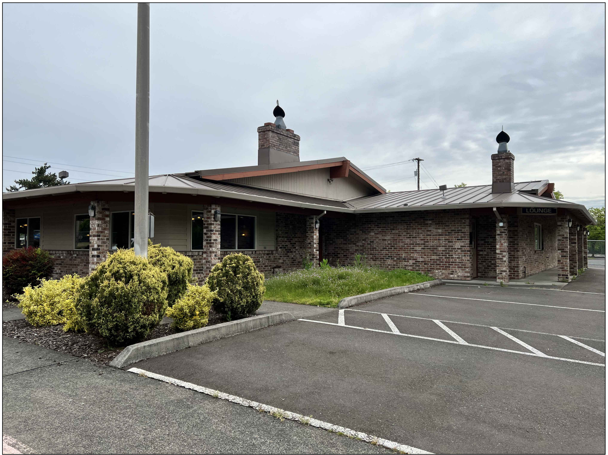
PHOTO 2- SW CORNER OF EXISTING BUILDING
