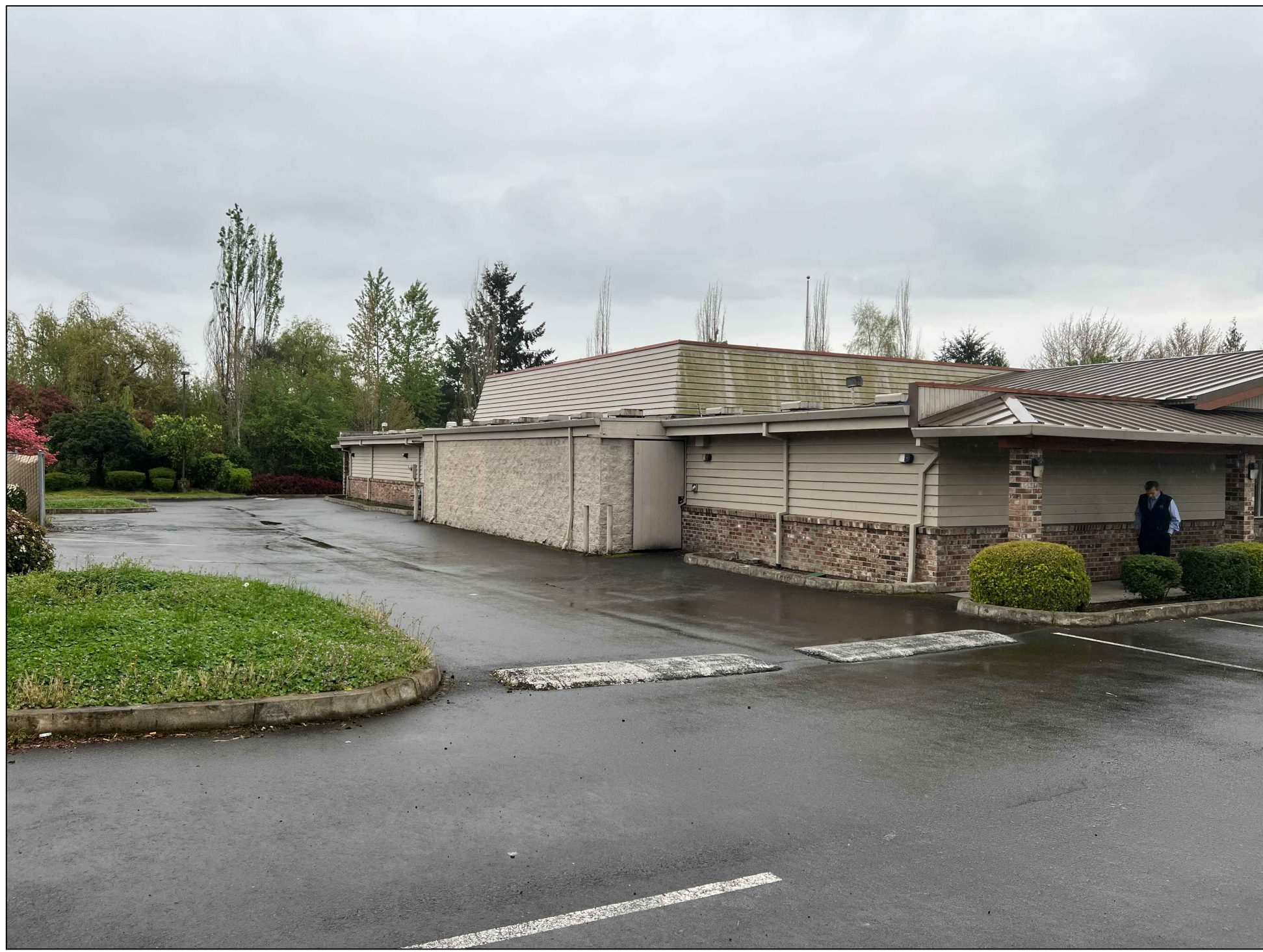
PHOTO 3- NE CORNER OF EXISTING BUILDING
