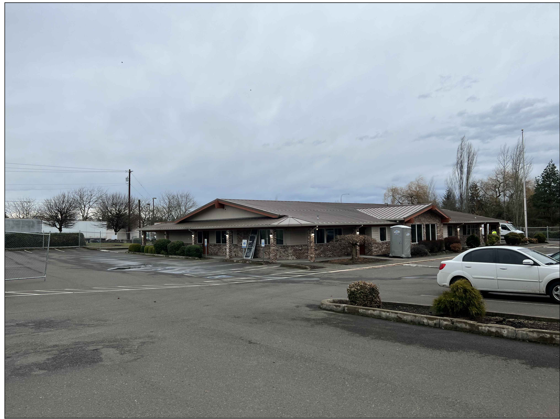
PHOTO 1- NW CORNER OF EXISTING BUILDING
