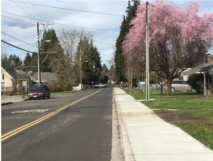
2017 Sidewalk Infill Project- Neals and Rossiter lanes
