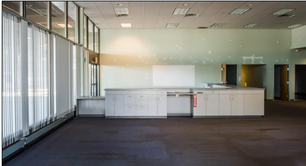
Day Center rehab in progress
