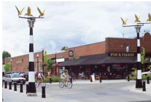
raised intersection with markers
