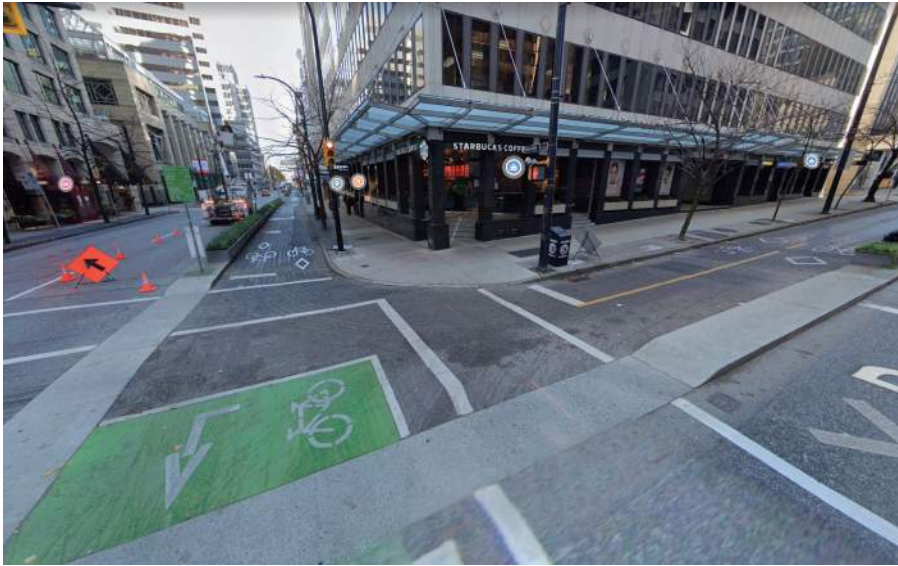
Turn box at 2-way cycle track intersection, Vancouver BC ('Copenhagen Left')
