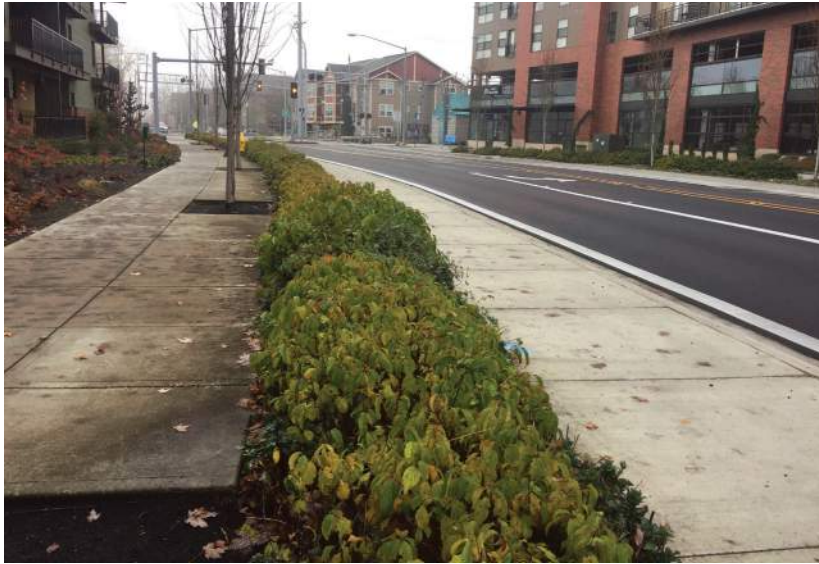
Adjacent to roadway, concrete, rolled curb
