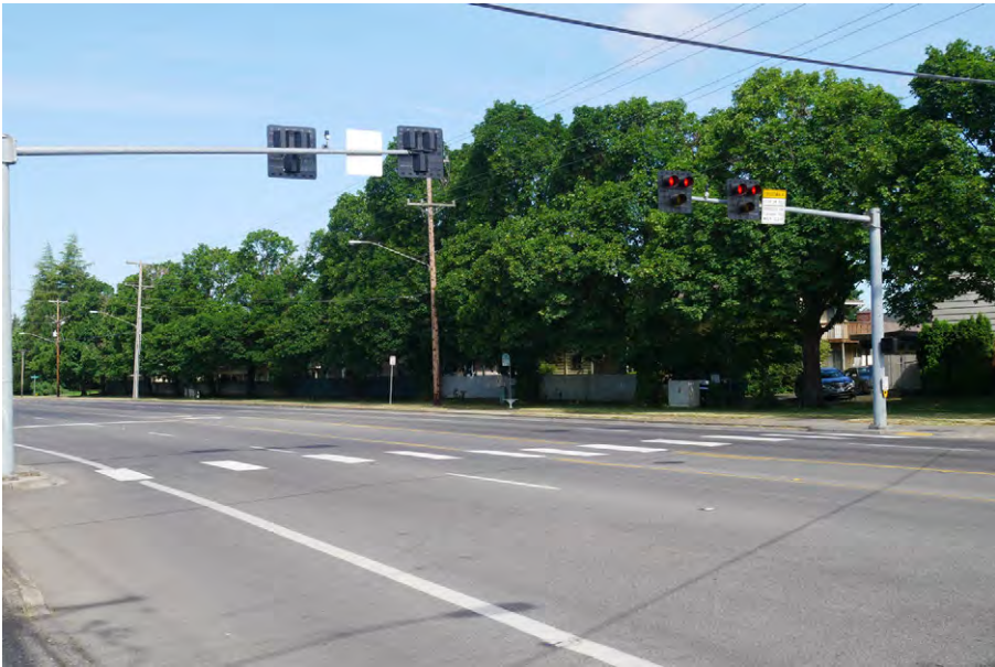
Pedestrian Activated Signal
