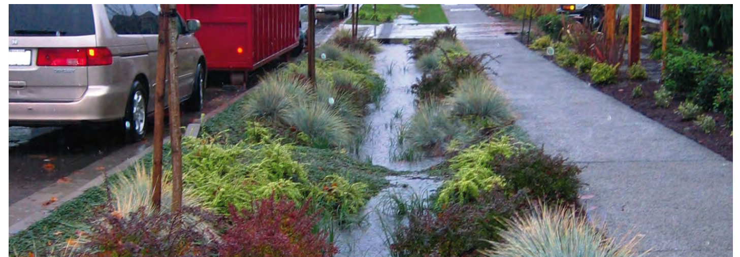
Stormwater Management in the Sidewalk
