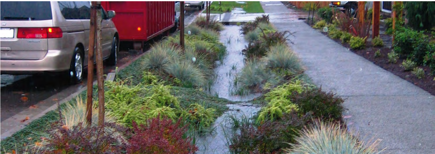
Stormwater Management in the Sidewalk
