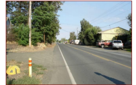
Shoulder bikeways are appropriate along wide roads where vehicles can avoid passing close to bicyclists
