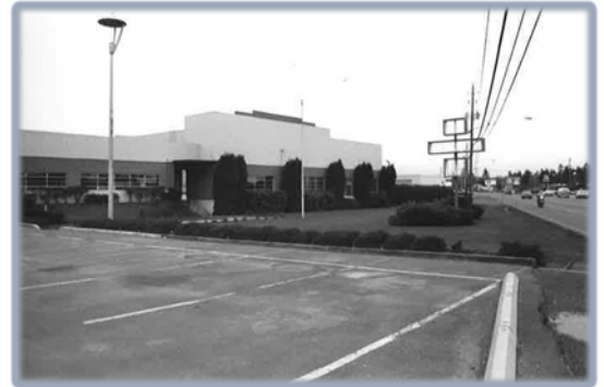
PW Ops Center Project - 3
