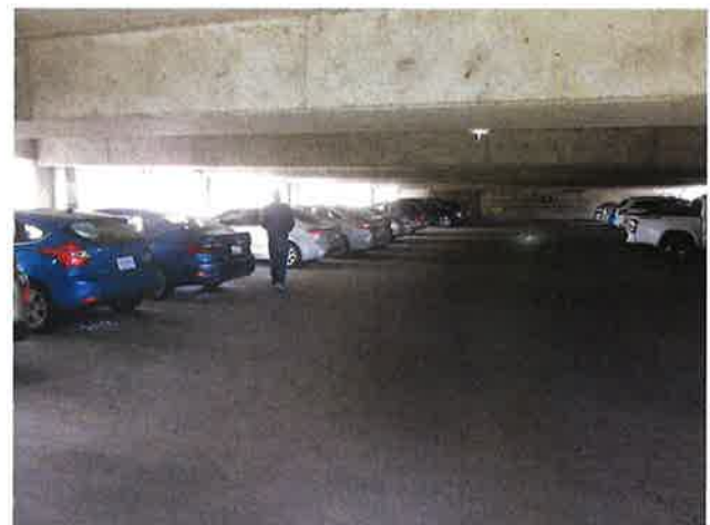
2 ND LEVEL SPACES ON RAMP UP FROM 1 ST LEVEL
