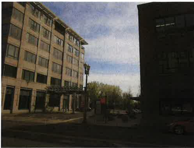
OVERVIEW OF SUBJECT IN DISTANCE AT LEFT (PAST COLUMBIA BANK BUILDING)
