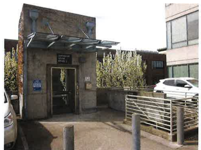
ELEVATOR AND STAIRS ON 3 RD LEVEL
