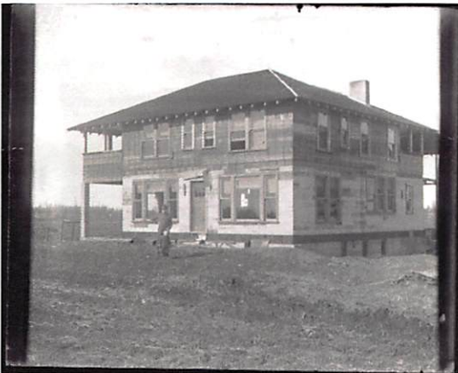
The view is towards the northwest. Photograph courtesy of Jennifer English. The Eclectic house under construction in 1917. 1917
