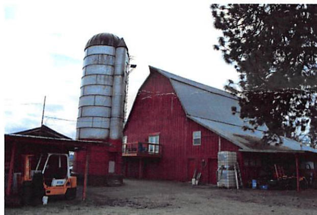
The view is towards the southeast. The north elevation of the 1915 barn (right), the circa 1970s silo (middle, Non-Contributing Feature 10) and circa 1970s machine shed (left, Non-Contributing Feature 9). 2014
