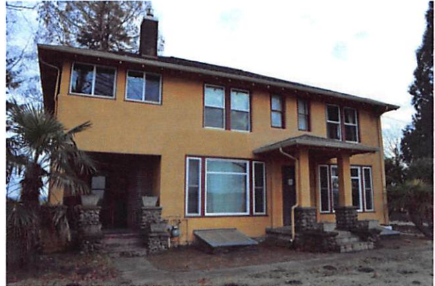
The view is towards the north-northeast. The south facade of the 1917 house (Contributing Feature 1). 2014
