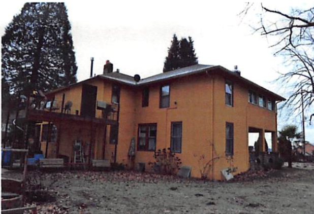
The view is towards the southeast. The west and north elevations of the 1917 house (Contributing Feature 1). 2014
