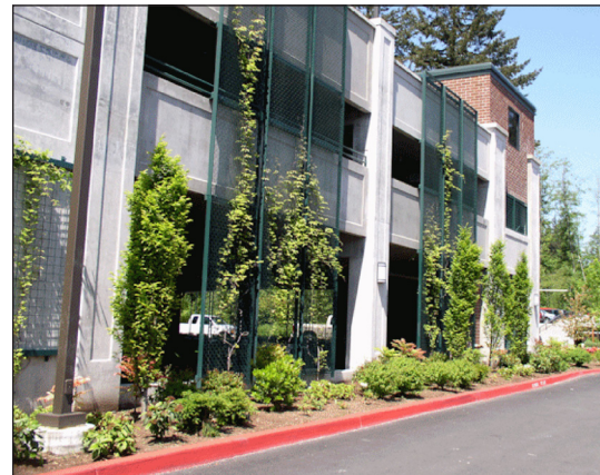
Figure 27. A good example of parking garage screening.
