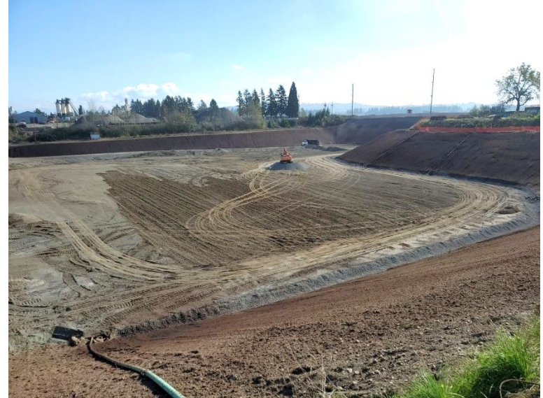
FROM THE WEST SLOPE LOOKING EAST
