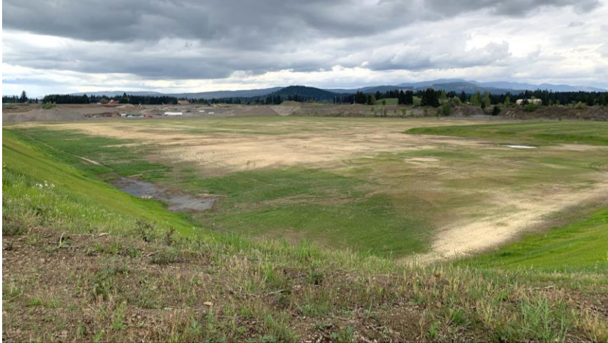
FROM SOUTHWEST CORNER OF PROPERTY LOOKING NORTHEAST
