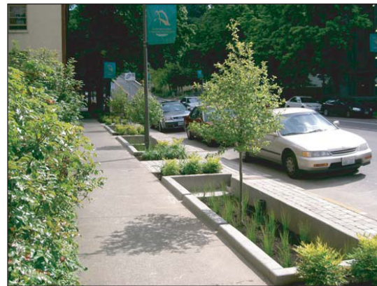
Figure 21. Example of rain garden.
