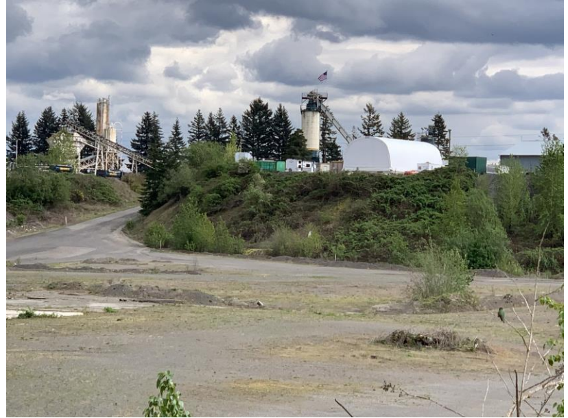
ASPHALT PLANT TO THE EAST OF HP PROPERTY
