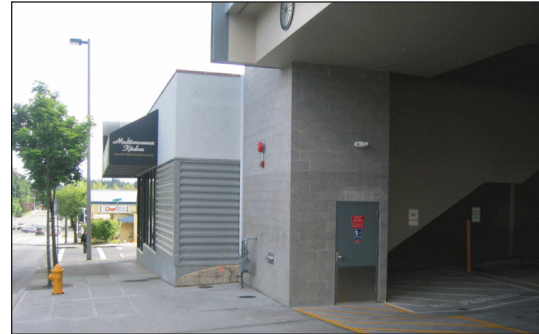
Figure 16. Avoid exposed utility meters like this.
