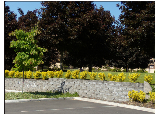
Figure 46. Example of retaining wall.
