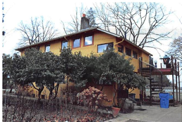
The view is towards the southwest. The east and north elevations of the 1917 house (Contributing Feature 1). 2014
