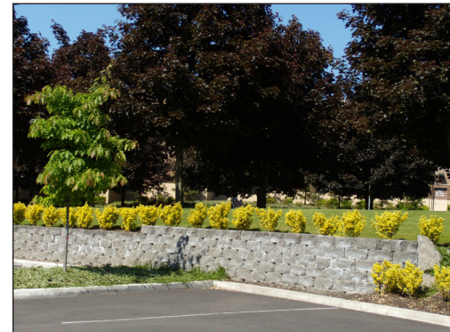
Figure 46. Example of retaining wall.
