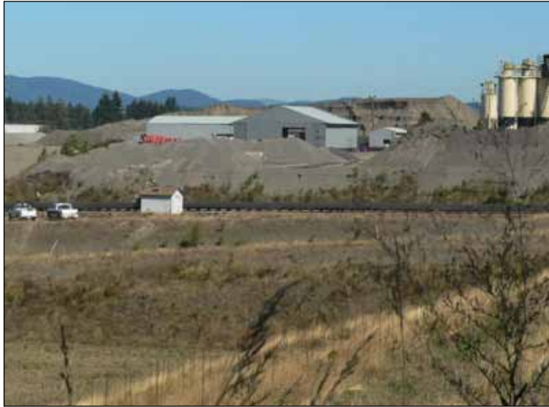
Existing gravel processing
