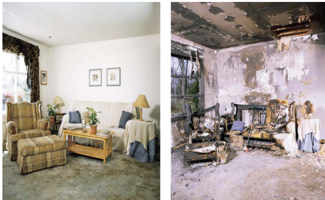
Figure 4. Fire Damage with and without Fire Sprinklers
