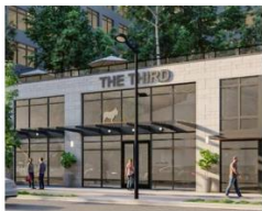
CLADDING - BUILDING ENTRY RECESS B.O.D. EQUITONE, INTEGRAL COLOR PREMIUM FIBER CEMENT PANEL - OFF-WHITE
