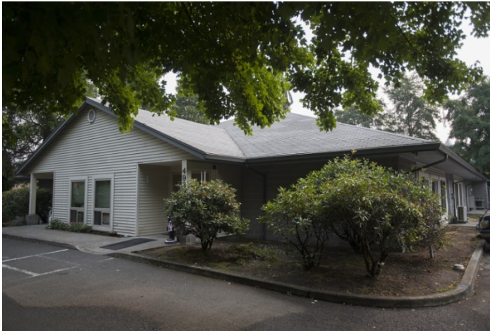
Valley Homestead Shelter
