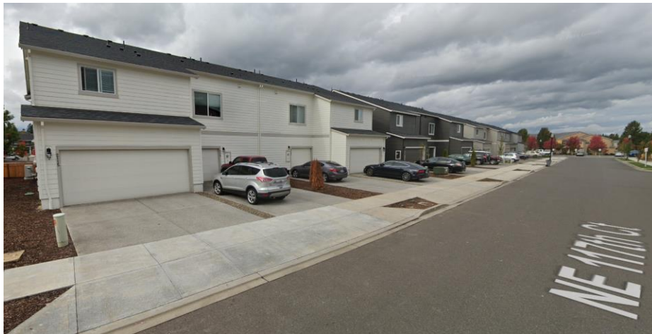
Four Seasons 4-plex on NE 117 th Court
