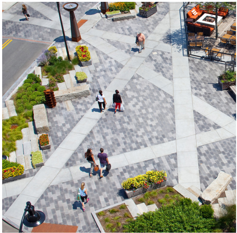
BRICK PAVING + CONCRETE BANDS
