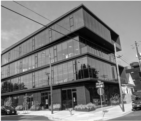
DON'T Create buildings with 100% glass curtain wall.
